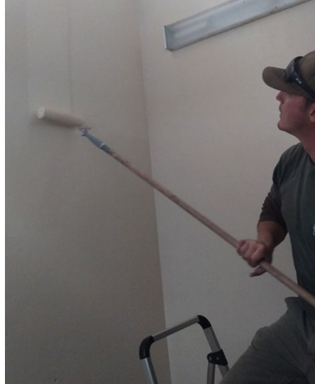
Ranger Hatton Painting VC Restroom Walls
