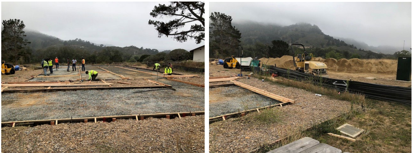
Placement of the Multi-Purpose Event Pad
