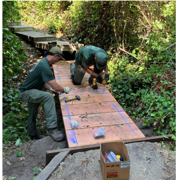
Construction of New Puncheon
