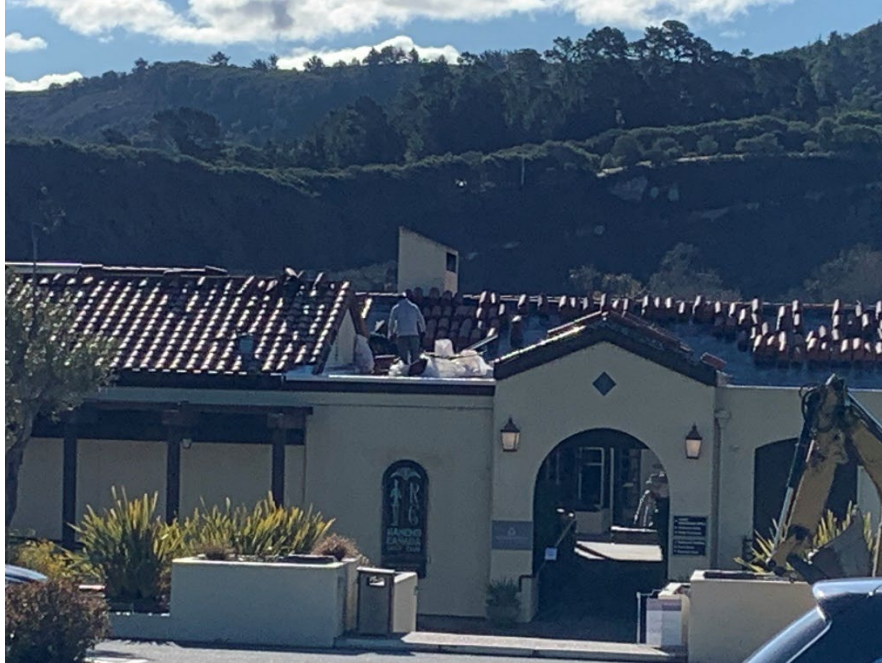
Tile roofing replacement over MPRPD's offices
