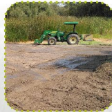
Frog Pond dredging to maintain pond catchment
