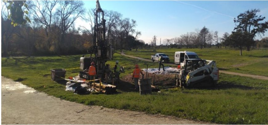
Cascade Drilling on-site at PCRP
