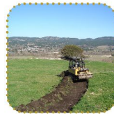
Palo Corona new trail construction
