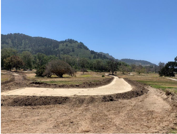
Permeable decomposed granite trail
