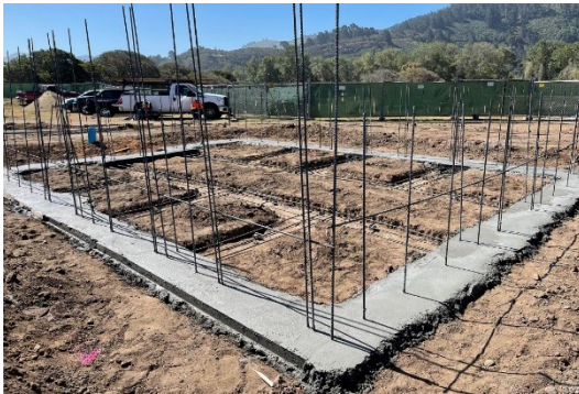
Restroom building foundation
