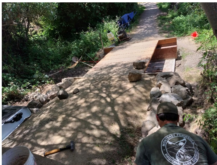
Rangers Hatton and Jared construct ramp approaches
