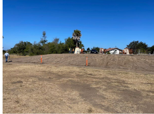
Repurposing excavated soil to create future main gate trail access
