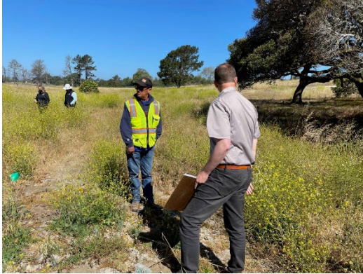
Contractor and Civil Engineer reviewing field layout of piping
