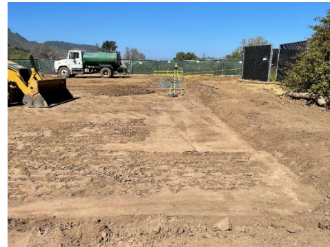
Multipurpose pad excavation
