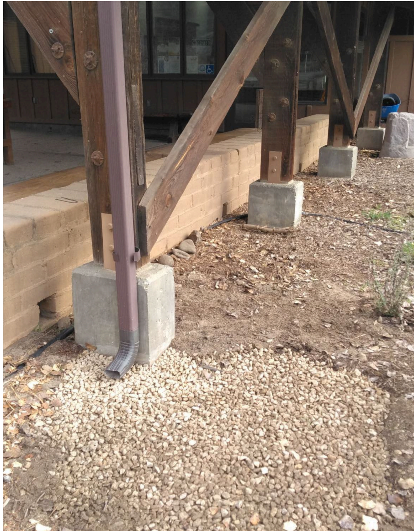
Drainage basin beneath gutter downspout at GRRP VC
