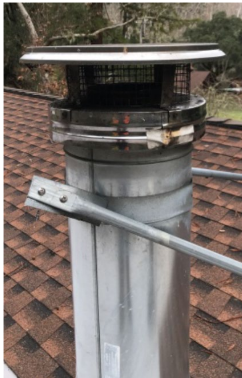
Spark arrester at Ranger Station
