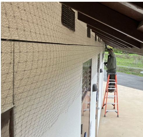
Exclusion netting installation
