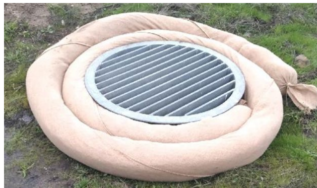
Biowaddle around drainage inlet
