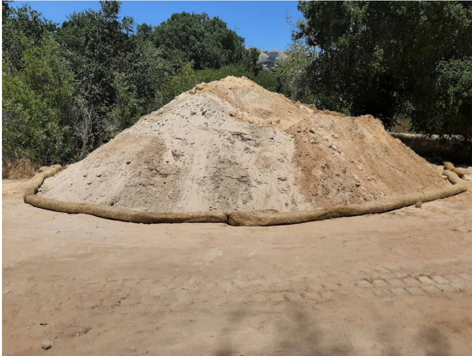
Stockpiled sand for next flood event
