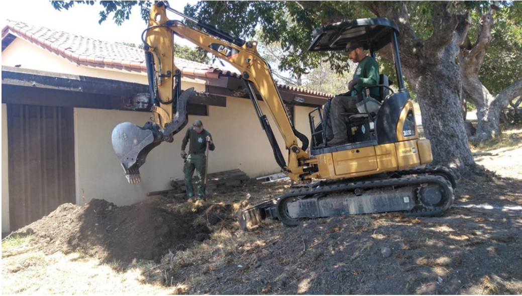
Rangers Jake and Jared dig the trench for electrical service
