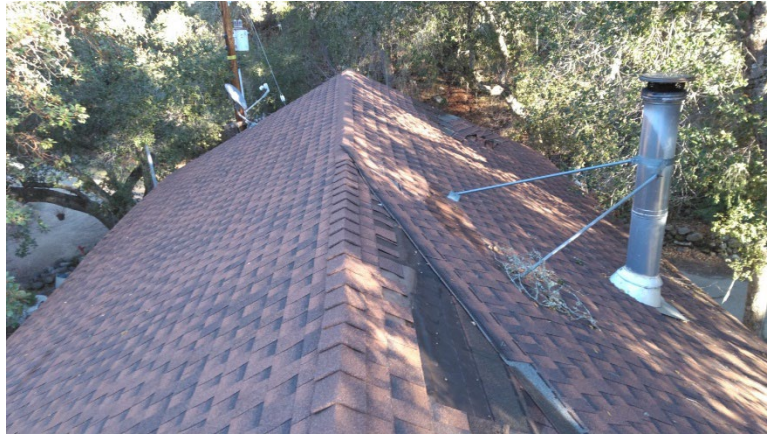
CCC Apartment Roof
