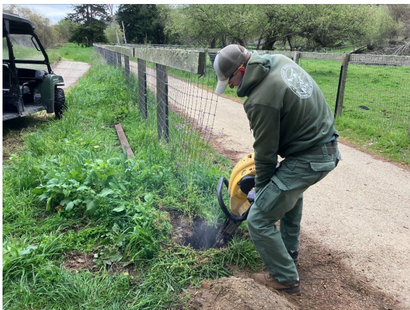
Ranger Martens jackhammering old concrete
