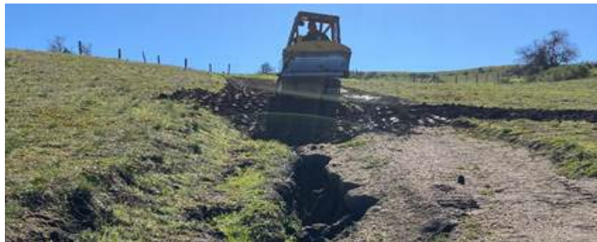
SWECO repairing damaged road segment
