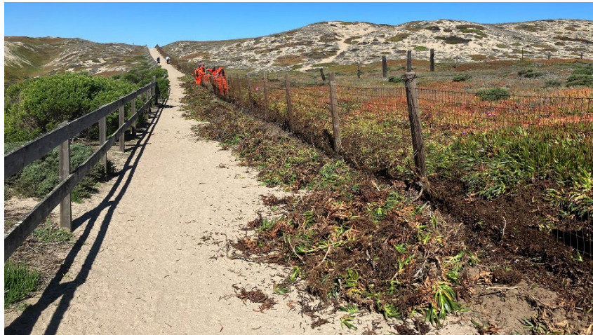
Gabilan Crew removing iceplant at MDP entrance trail
