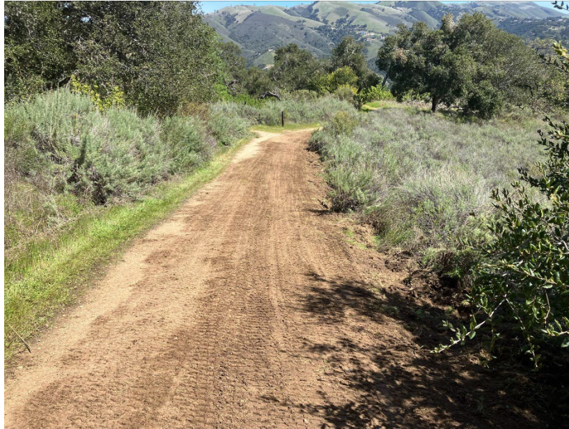
Finished section of Oakview Trail
