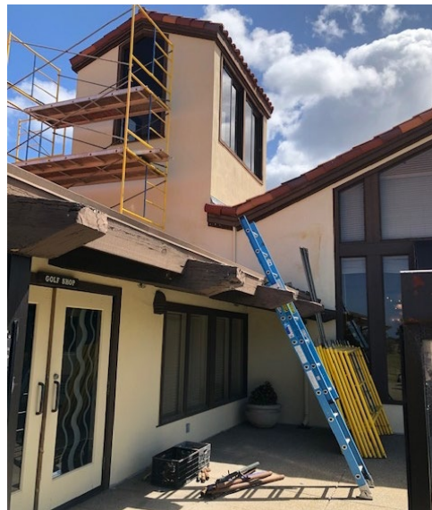
New Window Installation
