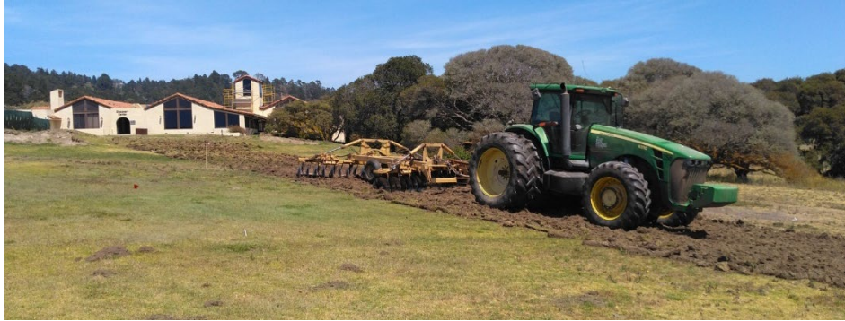
Contractor Prepping Trail Alignment by Removing Turf Grass
