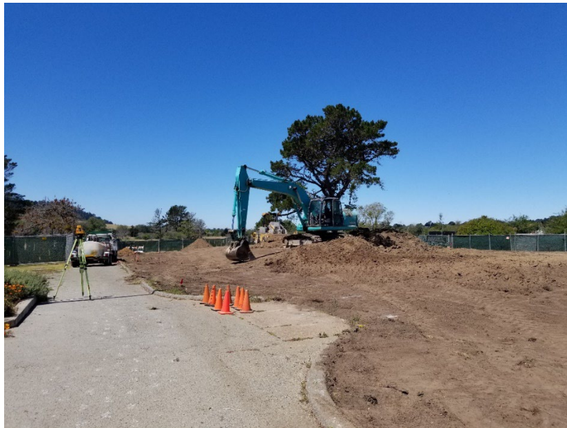
Restroom Pad Excavation
