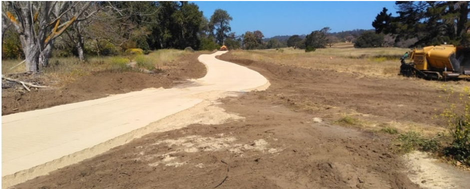
Permeable Decomposed Granite Being Laid and Compacted
