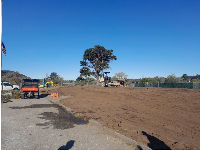
Fencing and Signage Installation
