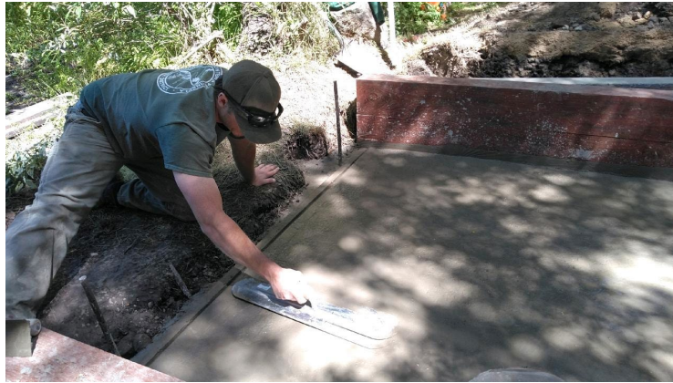
Ranger Vandervort Finishing Concrete Spillway
